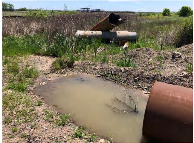
Photo 2: CHFR-1 – Unvegetated pooling water in the PDA at culvert outlet.
