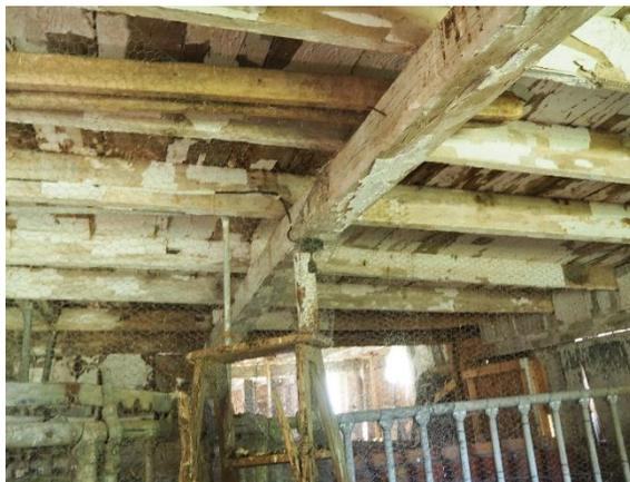
Plate 29: Hand hewn and machine cut timber
