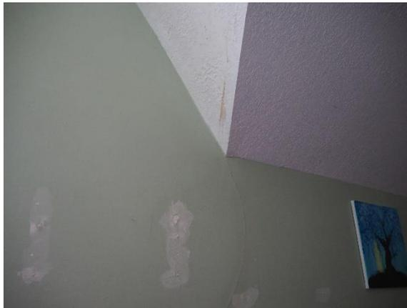
**Plate 34: Patched plaster cracks in second floor laundry room of rear unit**
