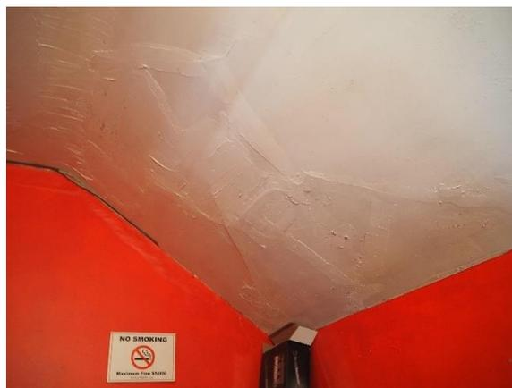
**Plate 32: Patched cracked plaster on second floor bedroom of front unit**
