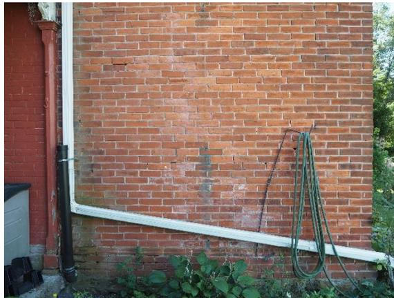
**Plate 38: Efflorescence and missing mortar on west elevation near entrance porch**
