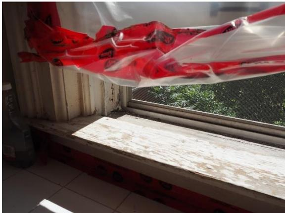
**Plate 33: Work paint on windowsill of second floor bathroom, front unit**
