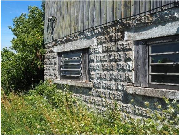
**Plate 41: Rusticated concrete block foundation with limited cracking**
