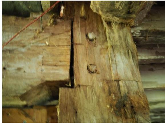
**Plate 44: Mortise and tenon construction with some separation**
