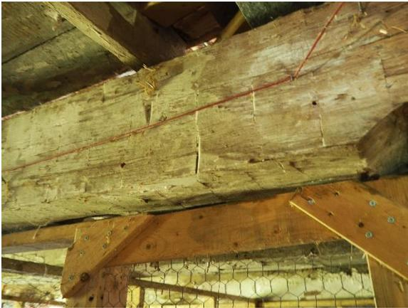
**Plate 43: Hand hewn interior beams showing little damage**
