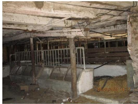
**Plate 41: Interior structural beam of questionable integrity**
