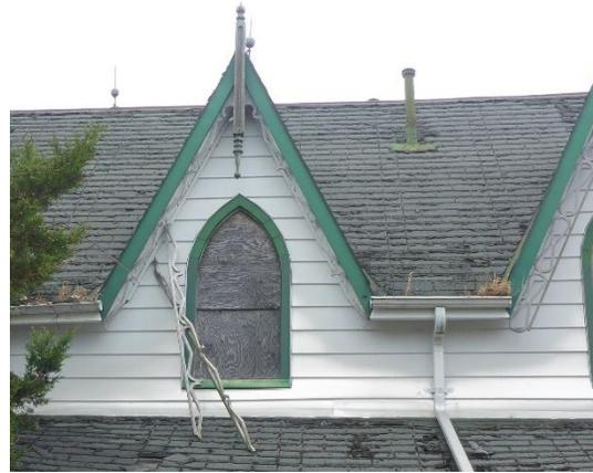
**Plate 29: Worn paint and damaged bargeboard**
