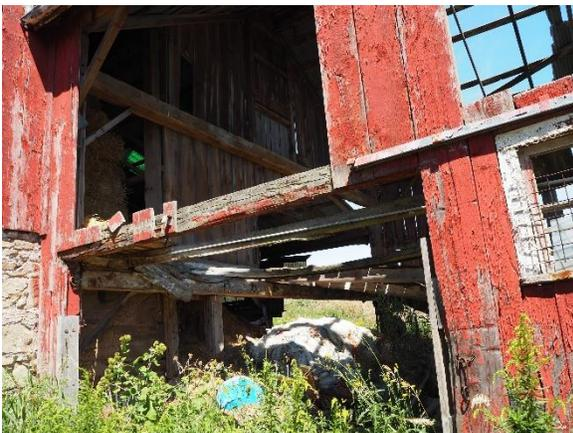
**Plate 27: View of partially collapsed roof and hand hewn beams**
