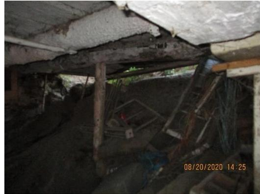
**Plate 39: Collapsed foundation wall**
