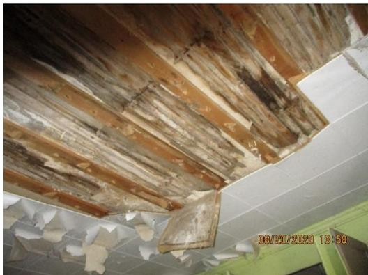
**Plate 34: Water damaged ceiling tiles**
