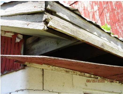
**Plate 40: Collapsing exterior structural beams**
