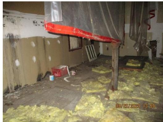
**Plate 33: Water damaged drywall and black mould**
