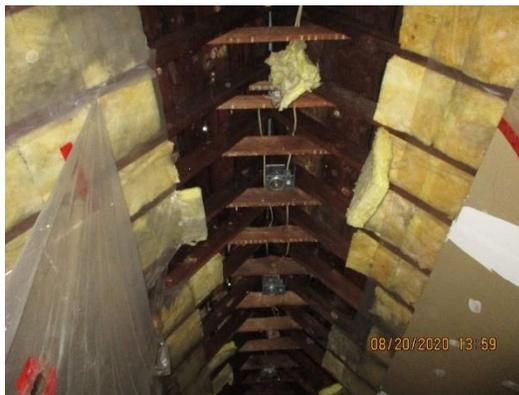
**Plate 35: Water damage from roof leak**
