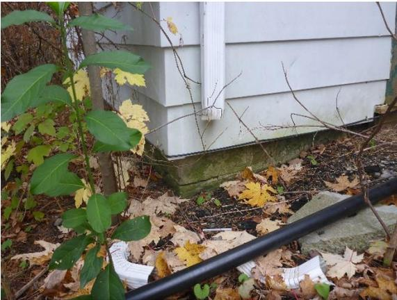
**Plate 30: Downspouts draining to foundation**
