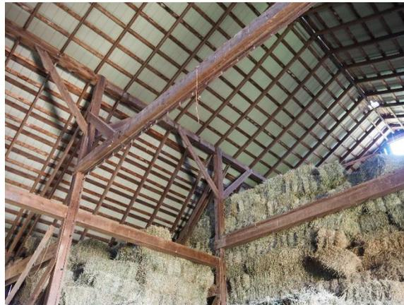
**Plate 26: Machine cut beams, posts, and joists**
