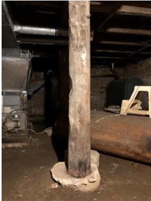
**Plate 33: Support post on concrete footing in the basement showing signs of water intrusion**
