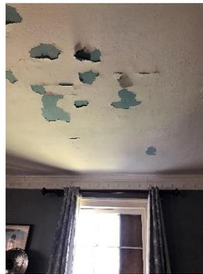
**Plate 30: Localized plaster cracks and peeling paint in living room**
