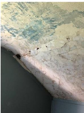
**Plate 31: Cracking plaster on upstairs ceiling**
