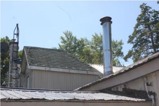
**Plate 27: Shingled portions of roof in poor condition, looking southwest**
