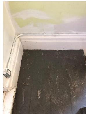
**Plate 17: Original floor moulding on first storey landing**
