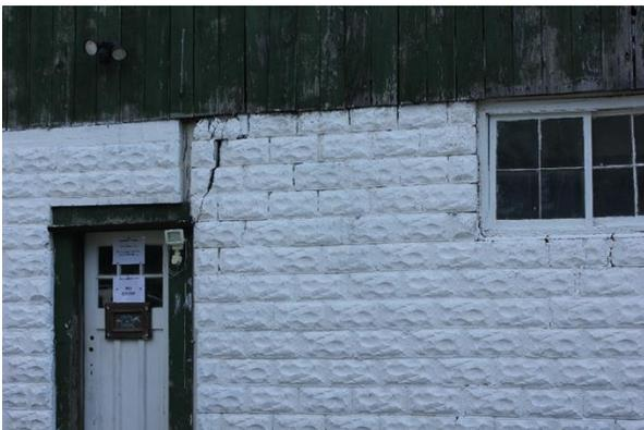
**Plate 34: Localized cracking in the concrete foundation of the barn, looking west**
