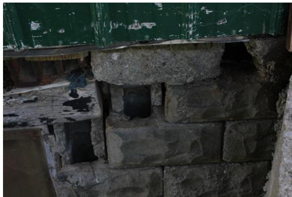
**Plate 35: Broken blocks supporting rotting wooden lintels**
