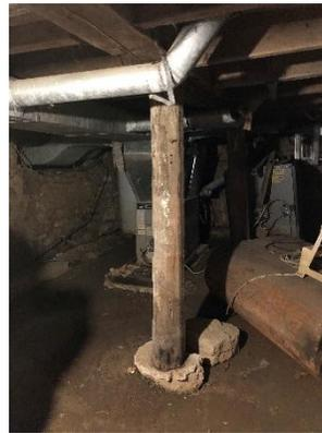
**Plate 13: Timber support beams on concrete footing**
