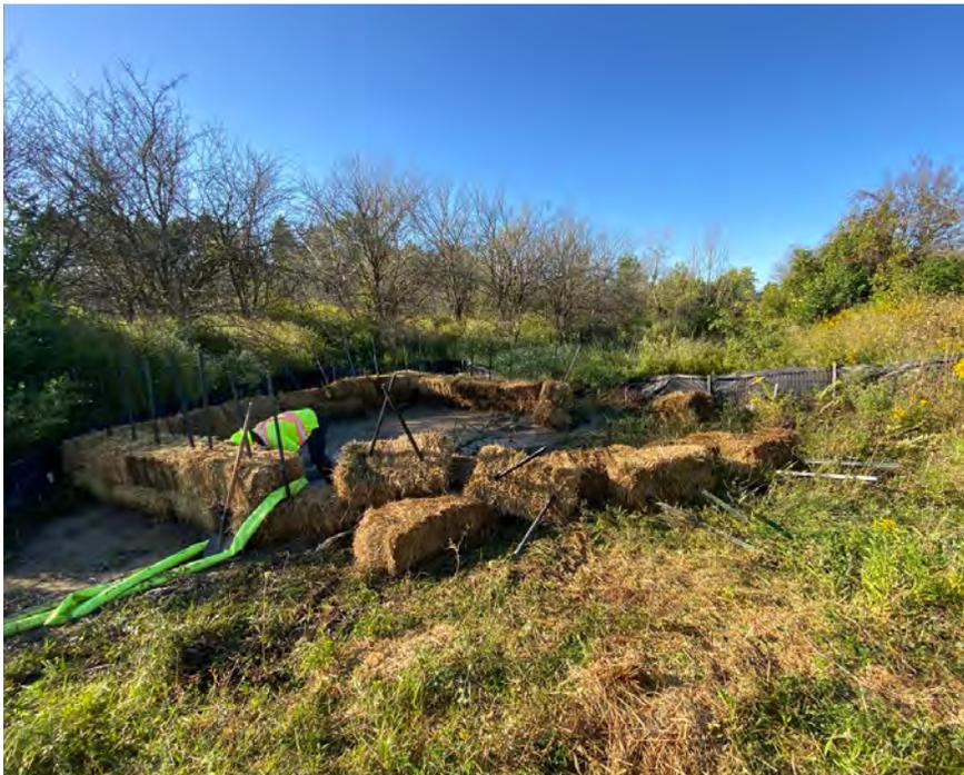
**Photo 1: Failed filter bag**
