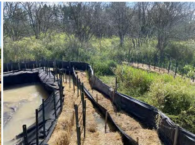
**Photo 5: Double silt fence with additional strawbales**
