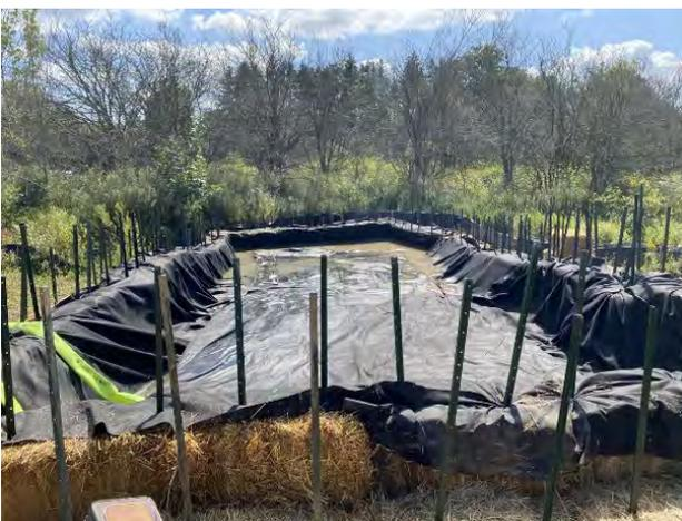
**Photo 6: Installed filter fabric liner and filter bag in sediment basin**
